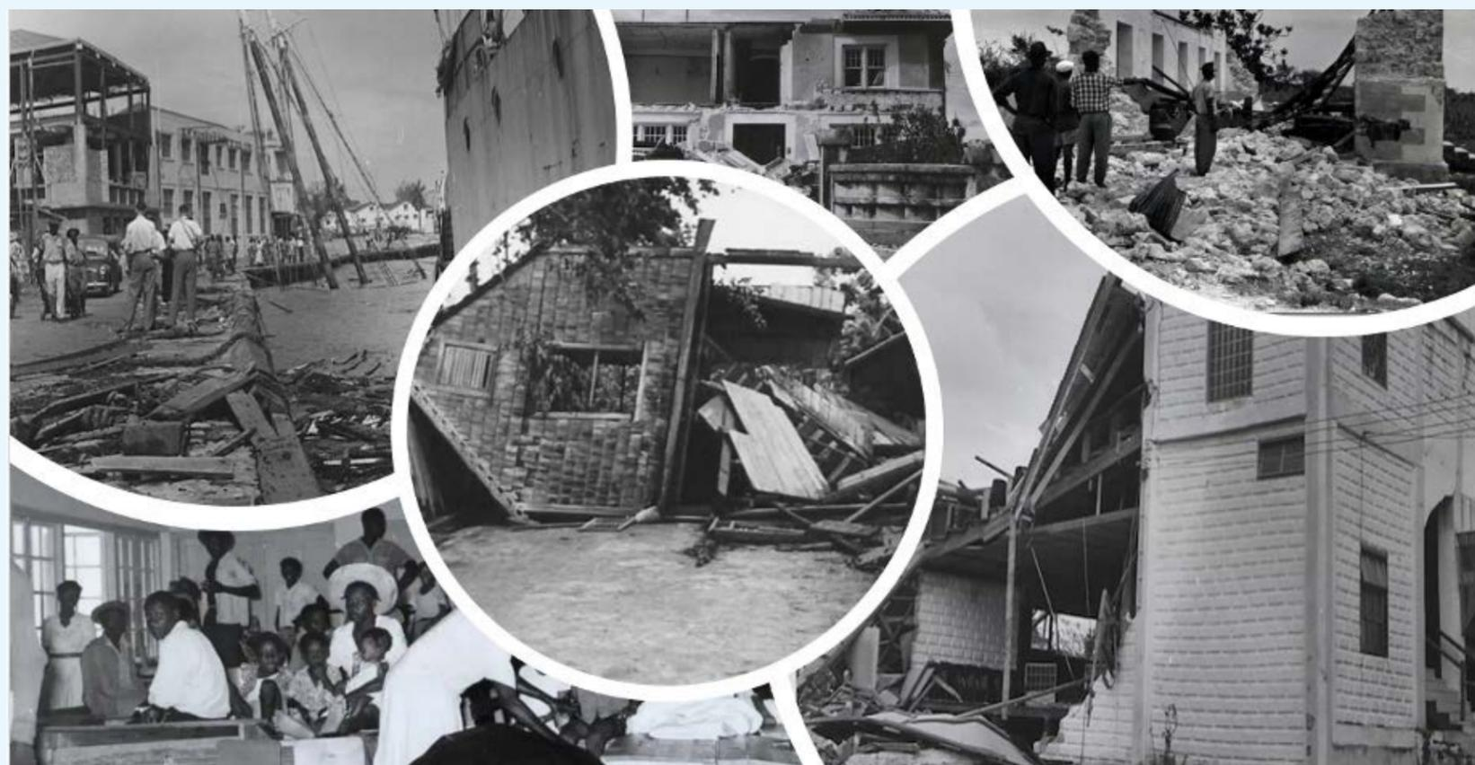
Figures B2: The extent of infrastructural damage posed by Hurricane Janet
