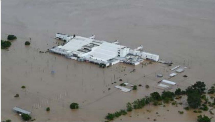
Flooding at San Pedro Sula airport
