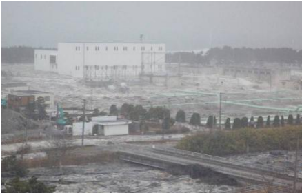
(Sewage plant struck by tsunami (Minami-Gamo Filtration Plant))
