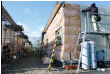
Heat insulator installation
