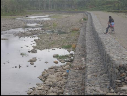
Gabions and dredging
