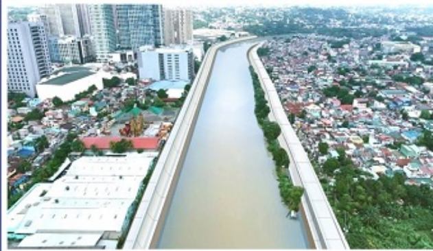
REVTMENTS AND FLOOD WALLS
