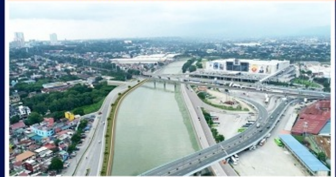
REVTMENTS AND FLOOD WALLS
