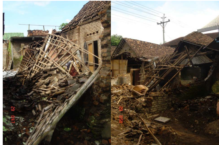
Condition of ruins in Bantul just after the quake in 2006
